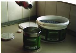
picture 1: mixing of resin + hardener component of Stop Stand.
