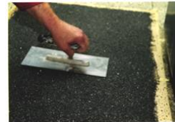
picture 4: compressing of the granules
